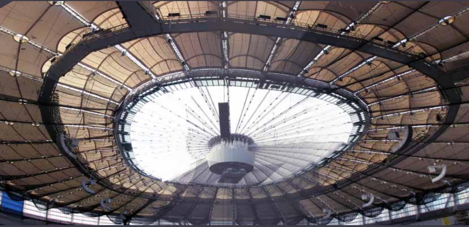
▲ PHOTO: 18,000 TONS OF STEEL AND 76,000 SQUARE METERS OF FABRIC WERE USED IN THE CONSTRUCTION OF THE NEW RETRACTABLE ROOF.
